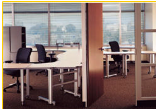
The Advanced Technology Development Center in Atlanta uses demountable walls throughout the incubator. These walls allow incubator staff to reduce or enlarge office suite size for new clients. Incubator clients also can move walls to create private offices within their suites.
